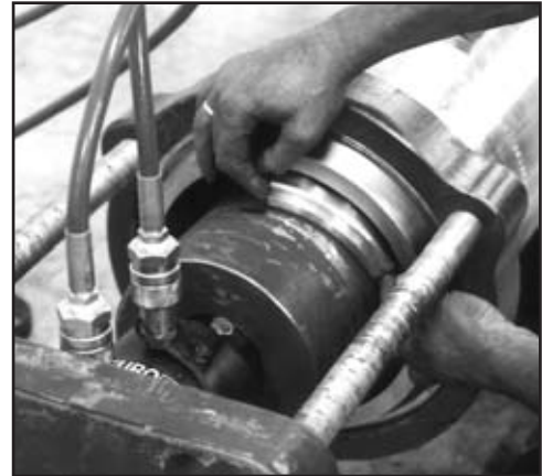
FIG. 131: INSTALL SEGMENT RING
